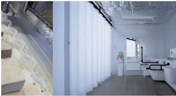
Fig. 6. Semi-transparent interior wall panel (photograph on the right by JUMPEI SUZUKI)
