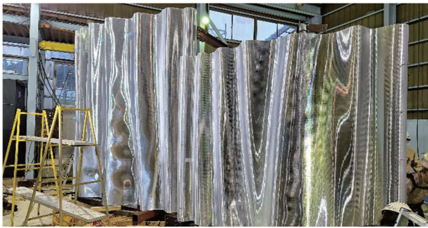
Fig. 10. Full-scale mock-up for construction assessment
